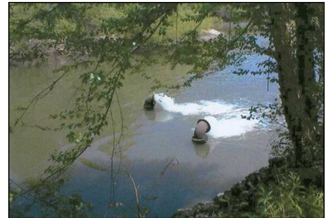
Combined Outfall Discharge to Ocmulgee River
